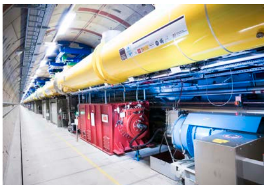
Fig. 1. 2.1km of accelerator modules in the tunnel of European XFEL (Hamburg)
